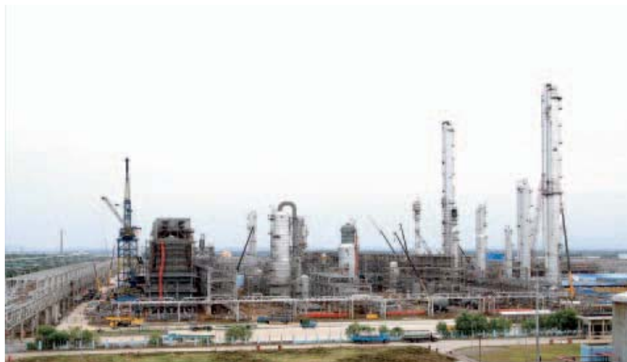
Figure 1: BASF chemical plant in China
