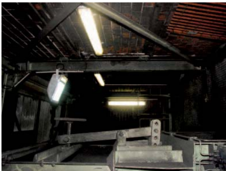
Figure 3: Special-purpose floodlights for metal-vapour lamps with a wattage of 250 and 400 W
