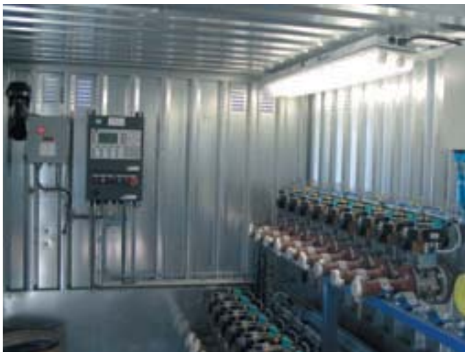
Figure 2: Container with filling plant and central control station for raw material delivery
