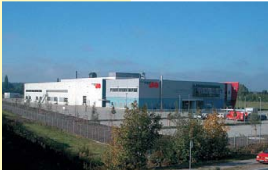
Figure 1: New plant building of the Jänecke + Schneemann company in Höver on the outskirts of Hannover, Germany
