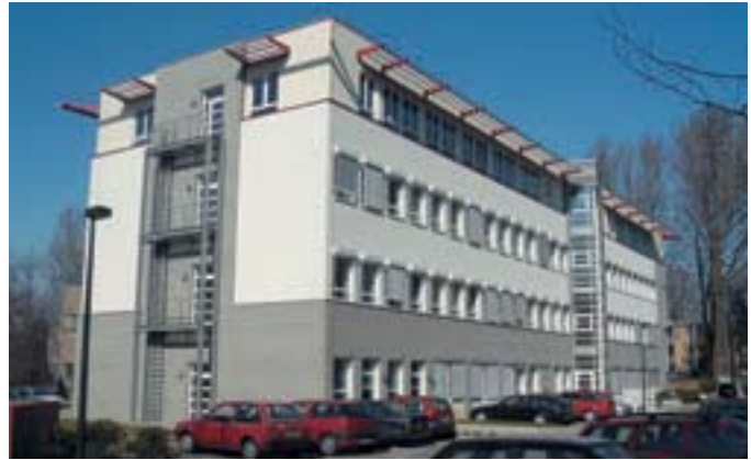
Figure 4: EXAM office and laboratory building in Bochum
