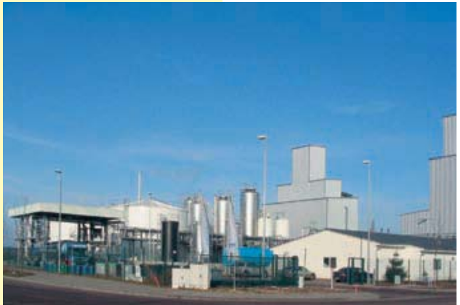
Figure 1: Biodiesel installation in Halle-Trotha
