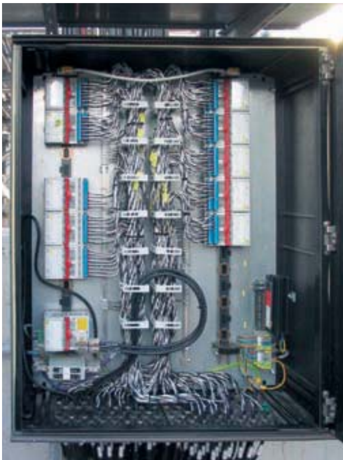
Figure 7: Station with Remote I/O Systems, with Power Module 9440, Digital Input Module 9470 and Analogue Output Module 9466
