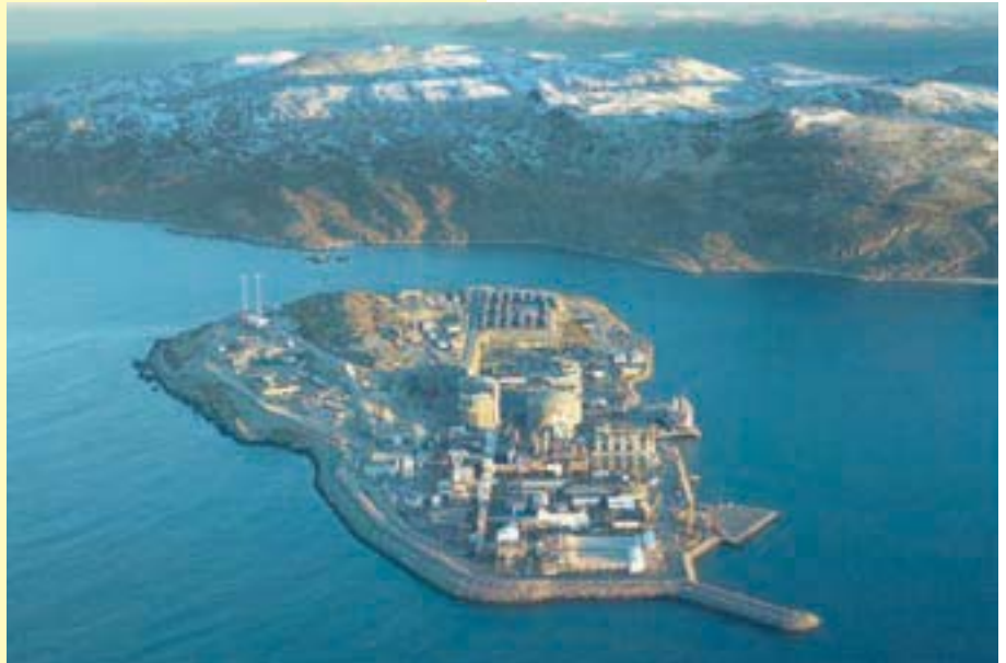
Figure 1: Gas liquefaction plant and LNG-terminal on the island Melkøya
