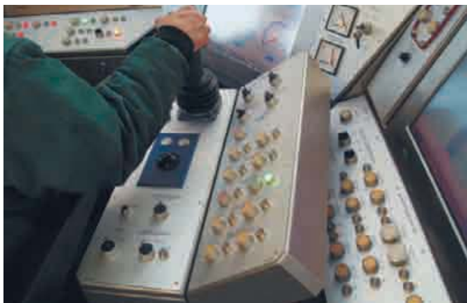
Figure 6: Controlling the increase in the length of the pipe using a joystick and other operator controls
