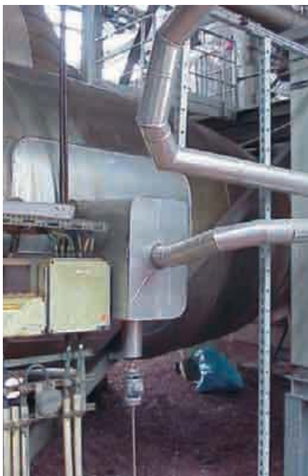
Figure 2: Sample taking and pipes of the steamheater. The sample must be heated exactly to 145 °C continuously
