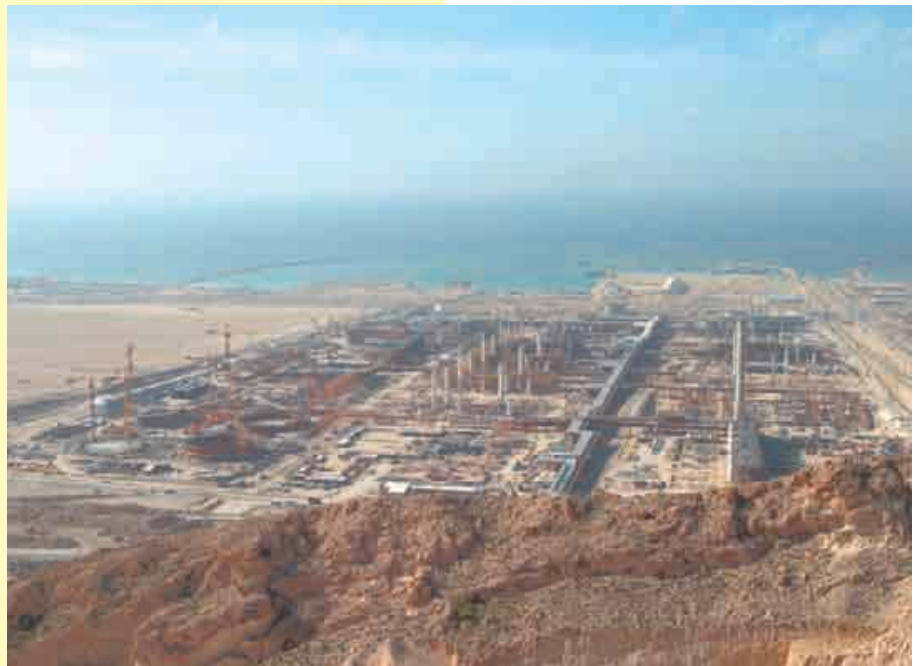
Figure 1: Building a gas processing plant in the Persian Gulf: South Pars
