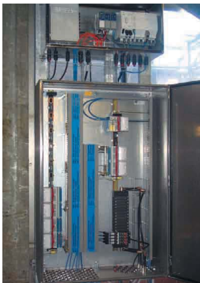
Figure 2, top: Controller in the housing with restricted breathing; bottom: Field station with built-in I/O systems and solenoid valves
