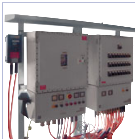
Figure 7: Control system in the flameproof enclosure system CUBEx
