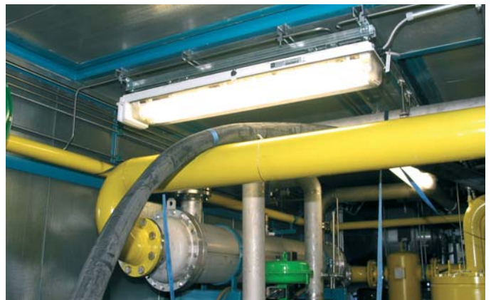
Figure 5: Emergency luminaire series EXLUX 6008
