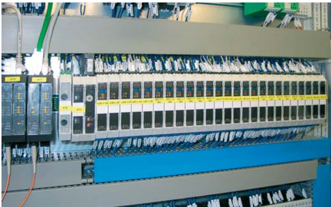
Figure 8: ISpac Isolators for safety-related signals
